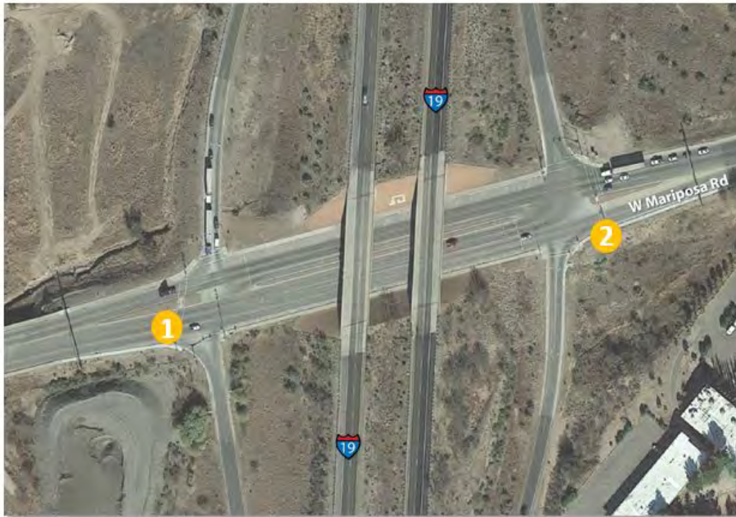
Figure 4-6 | Interchange at I-19 and W. Mariposa Road
