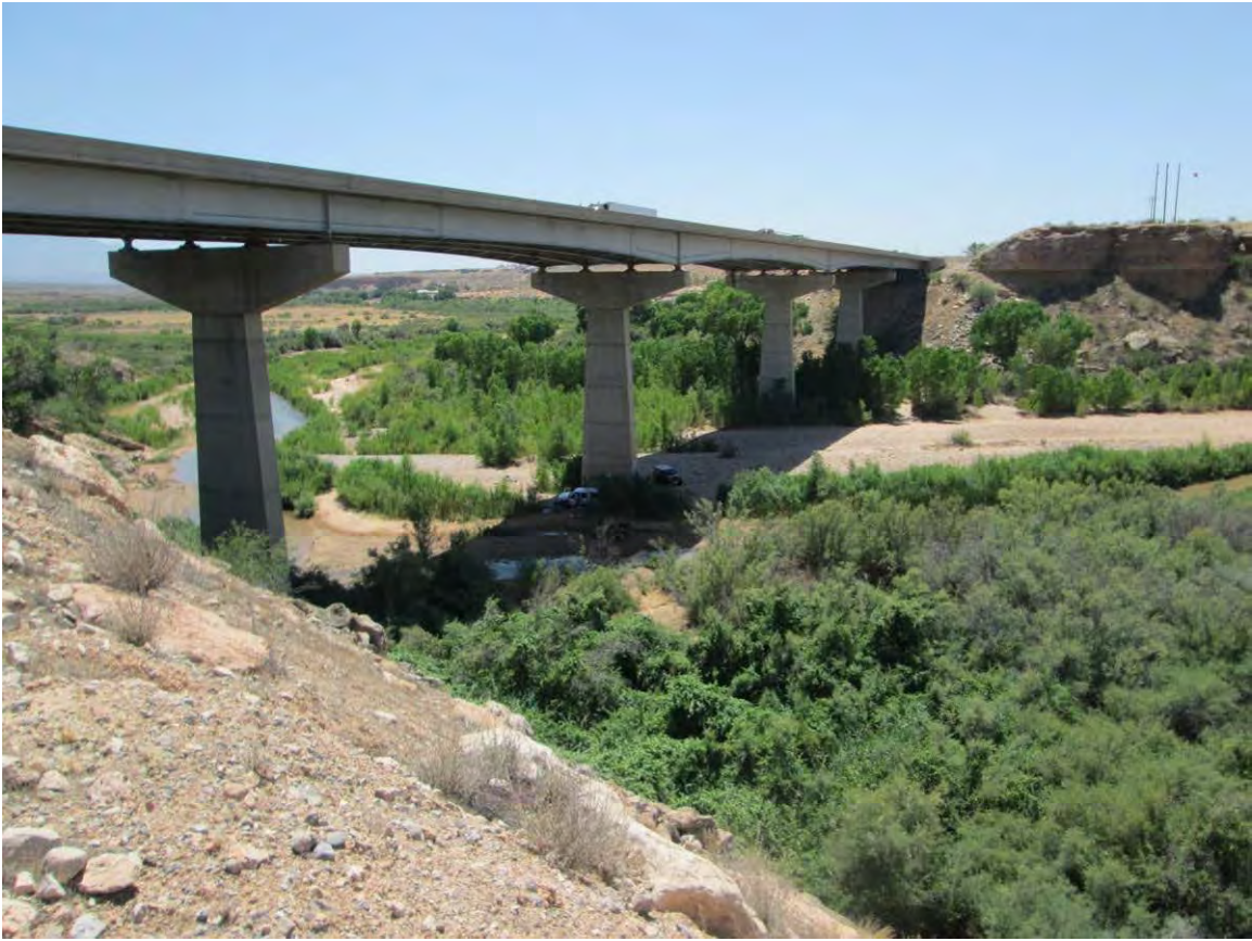
Photo 1. Northeast side of I-15 at Virgin River Bridge No. 1 (Bridge No. 1), looking southwest.
