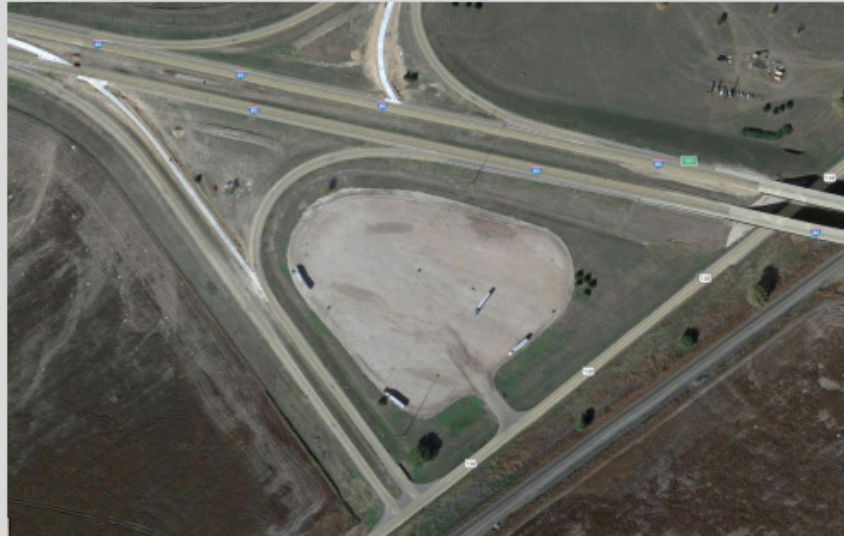
Figure 2-12: Low Cost Truck Parking Solution in Nebraska
