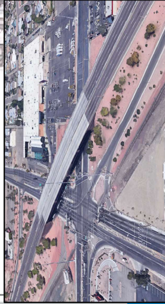
Example of elevated Grand Avenue at 43 rd Avenue
