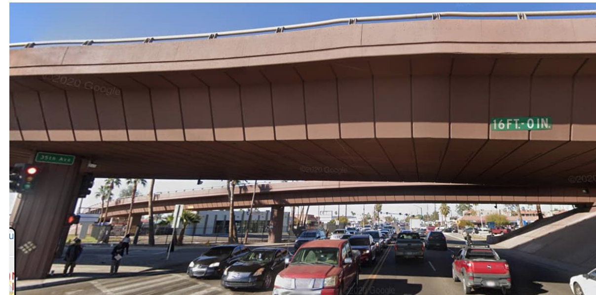
Figure 7 – Posted Minimum Vertical Clearance Over 35 th Avenue (Looking North)
