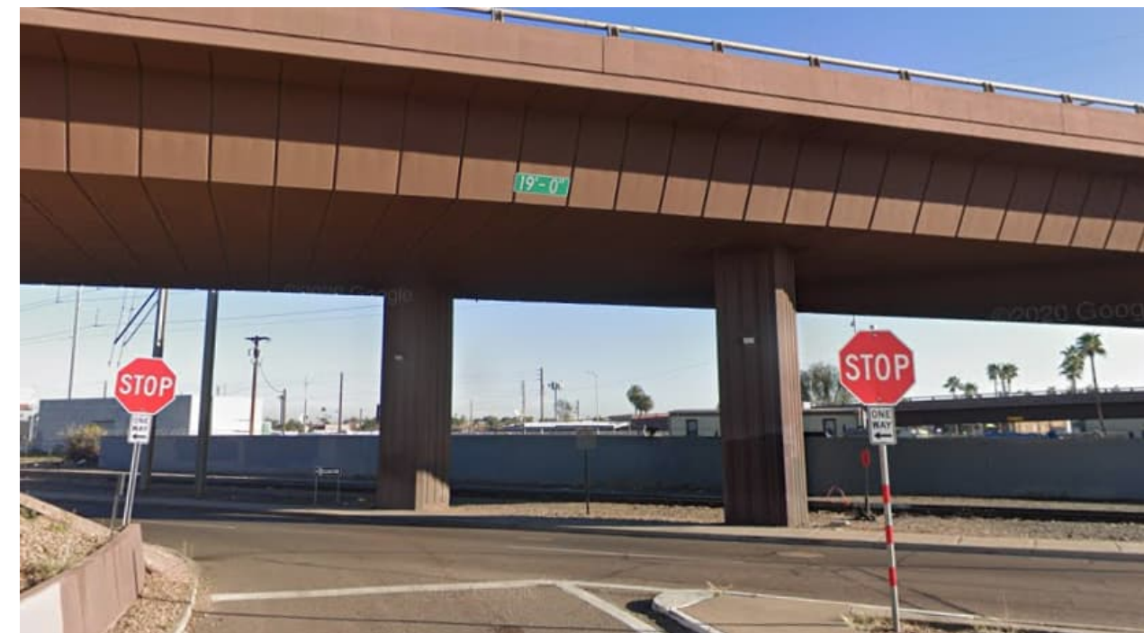
Figure 8 – Posted Minimum Vertical Clearance Indian School/US 60 Ramp Connections (Looking North)
