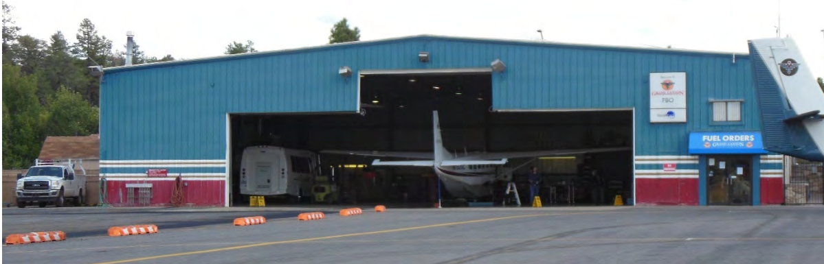
Grand Canyon FBO Hangar Source: Coffman Associates
