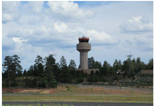
Rotating Beacon atop the ATCT
