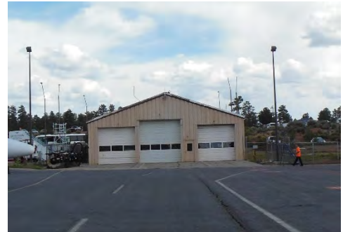
Previous ARFF Building Source: Coffman Associates
