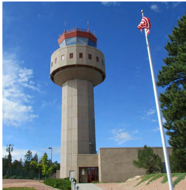
Airport Traffic Control Tower (ATCT)
