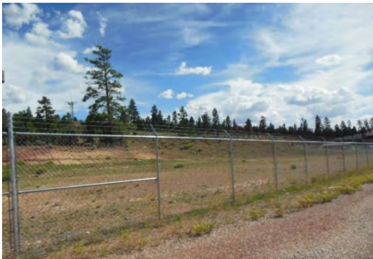
Perimeter Security Fence Source: Coffman Associates
