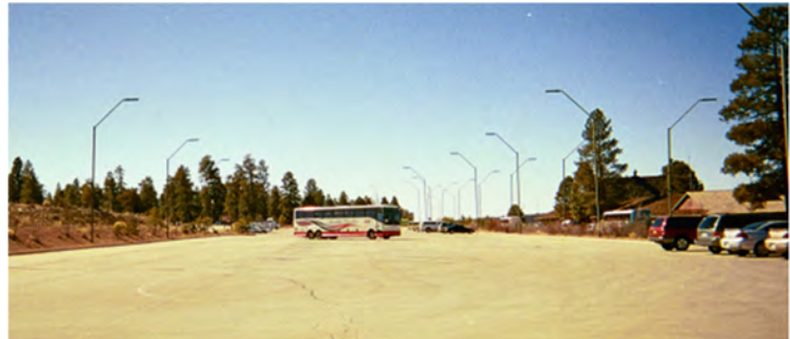
GCN Terminal Auto Parking Area (looking south)
