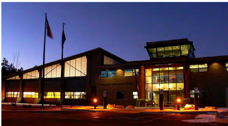
ARFF Station Source: Quest Energy Audit, 2016
