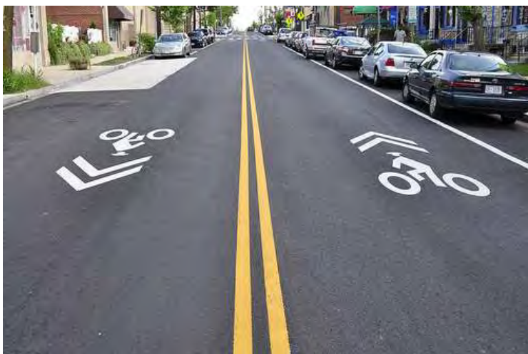
Figure 7-3 | Shared Lane Markings & Signage
