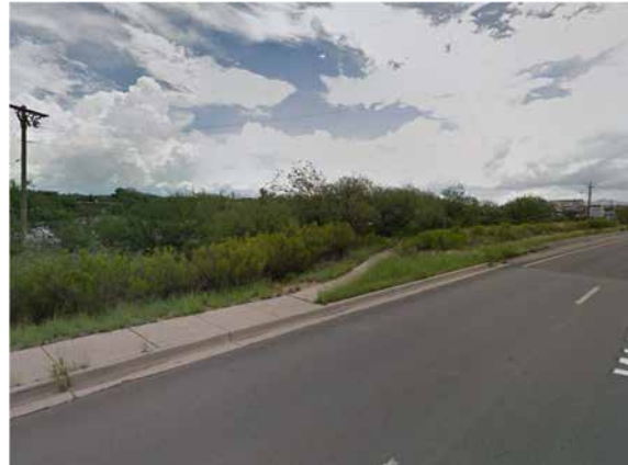
b) A segment of sidewalk west of Frank Reed Rd shifts away from Mariposa Rd and is hidden from view at times, presenting a possible personal safety hazard
