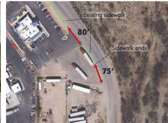
c) Several residential developments along Frank Reed Rd do not have sidewalk connections, such as this one on Placita H. Rivas
