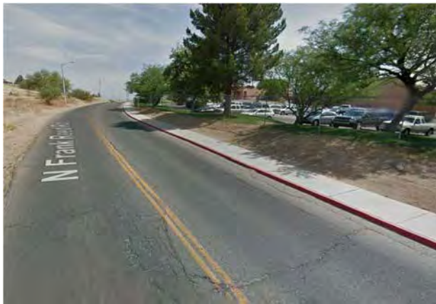
a) Most sidewalk along Frank Reed Rd is 5 feet wide and attached, and is in good condition
