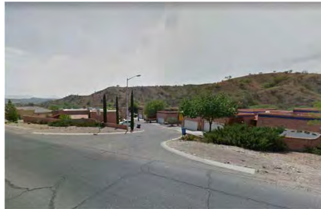
b) Several residential developments along Frank Reed Rd do not have sidewalk connections, such as this one on Placita H. Rivas
