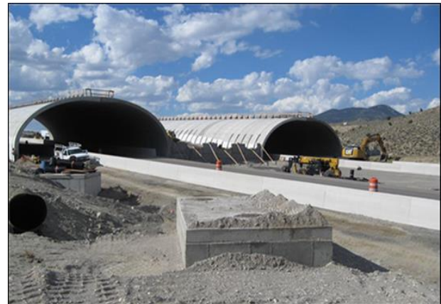
Figure 3- 73. Precast concrete arch overpass installation along I-80 in Nevada (NDOT) (photo).
