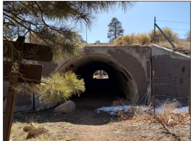
Figure 3- 9. Arizona Trail pedestrian arch underpass under US 89 near the junction with the Townsend-Winona Road (MP 420.7).
