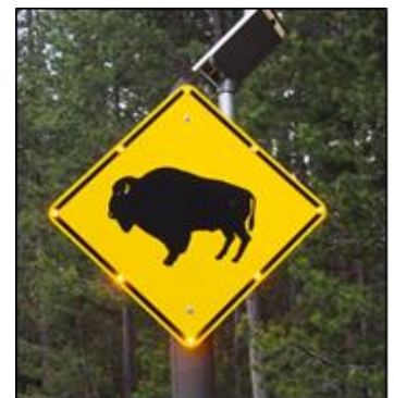
Figure 3- 87. Solar-powered motorist alert sign with LED flashers at a high-incidence bison collision zone in Yellowstone National Park. Such signage is especially effective at nighttime hours when many WVCs occur.
