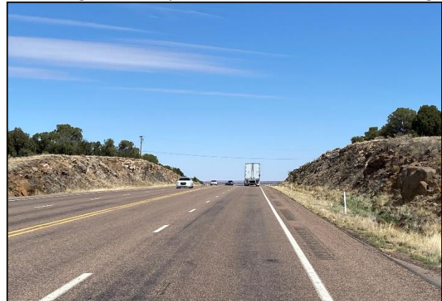
Figure 3- 48. Suitable site for a drop-in overpass at SR 77 MP 350.2 where the highway has already been widened to 4 lanes.
