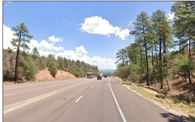
Figure 3- 79. Typical stretch of SR 260 Hotspot #10 between Payson and Star Valley.
