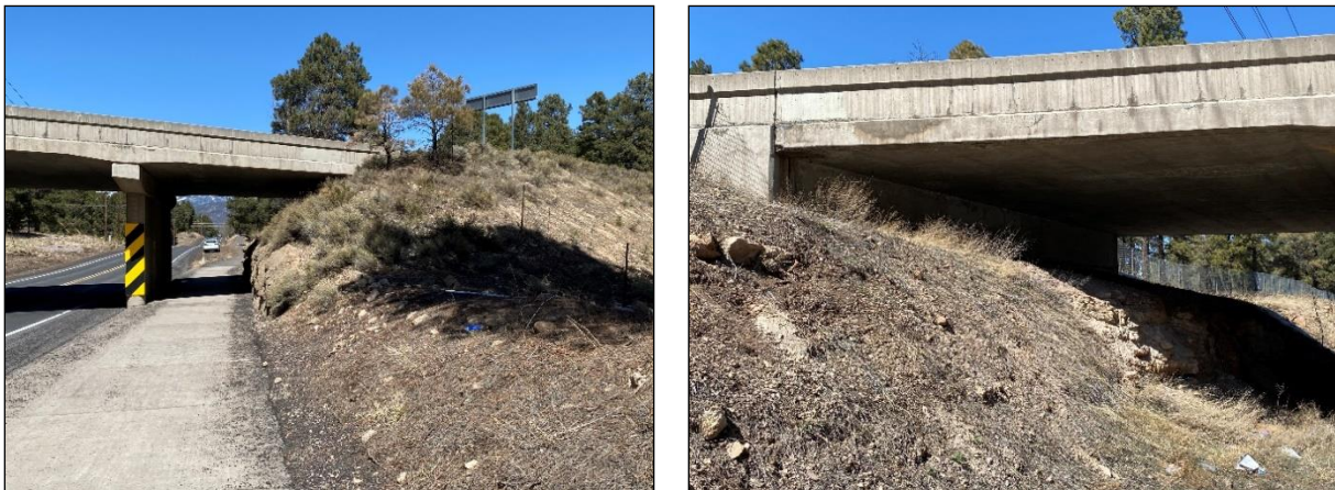
Figure 3- 40. The steep eastern bridge side slopes at the WB I-40 Lone Tree Road underpass with an adjacent urban trail (left) which limit wildlife passage through the structure. Passage could be enhanced if the side slopes were partially excavated to resemble the western side slopes (right) where animals could more readily pass under the bridges (right).
