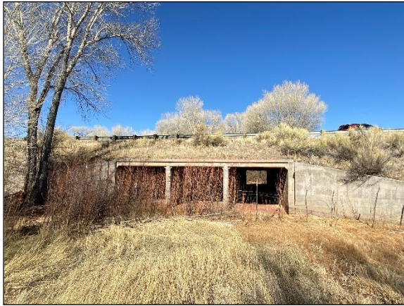
Figure 3- 46. Three-barrel CBC drainage structure where Show Low Creek crosses SR 77 (MP 354.4), the most suitable of any structures along Hotspot #4 for wildlife passage.
