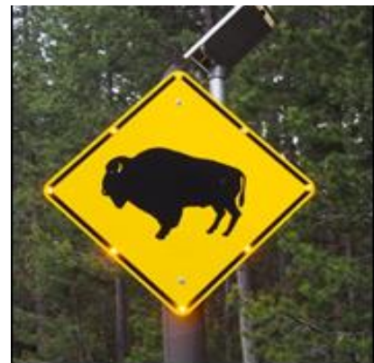
Figure 3- 52. Solar-powered sign with LED flashers at a high-incidence bison collision zone in Yellowstone National Park. Such signage is effective at nighttime hours when most WVCs occur.
