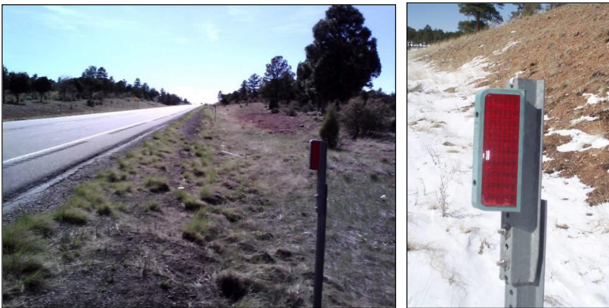
Figure 3- 61. SWAREFLEX wildlife warning reflectors along Hotspot #6, showing the installation location adjacent to the roadway to limit snowplow damage (left) and a closeup of a reflector mounted on a delineator post (right).
