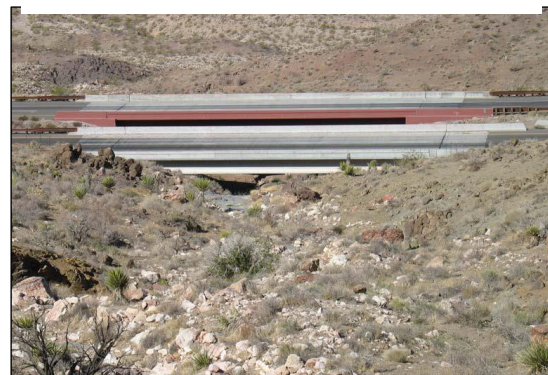
Figure 2- 15. SR 68 underpass at MP 10.8 which has very poor line-of-sight visibility affecting bighorn sheep use (photo from Bristow and Crabb 2008).
