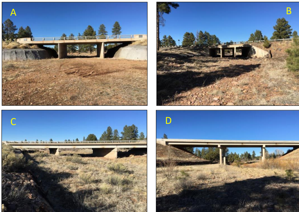
Figure 3- 60. Existing SR 260 structures suitable for wildlife passage: Pierce (A), Decker (B), Cottonwood (C), and Mortensen (D) wash bridges (from Gagnon et al. 2017).
