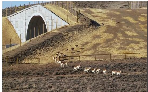
Figure 2- 26. Drop-in precast arch pronghorn overpass on US Highway 191 in Wyoming. Wildlife Conservation Society photo.
