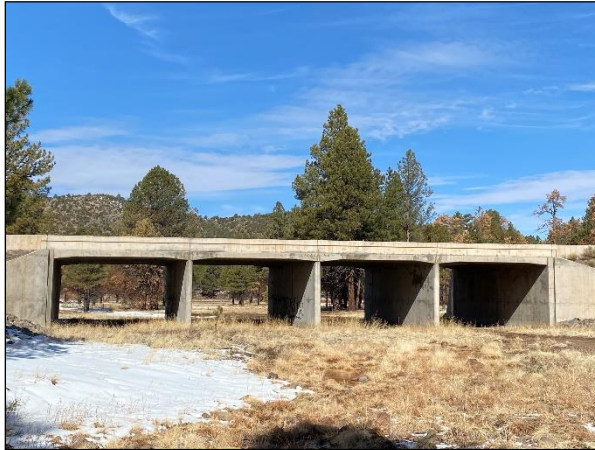
Figure 3- 99. SR 64 Cataract Canyon bridge located at MP 187.3 (left) and an individual barrel (right) suitable for accommodating elk and mule deer passage with wildlife fencing.
