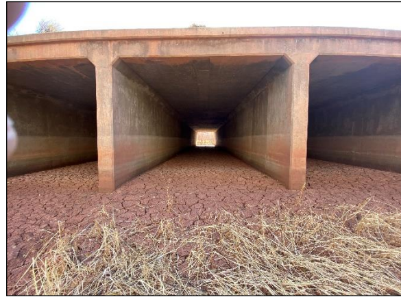
Figure 3- 46. Three-barrel CBC drainage structure where Show Low Creek crosses SR 77 (MP 354.4), the most suitable of any structures along Hotspot #4 for wildlife passage.
