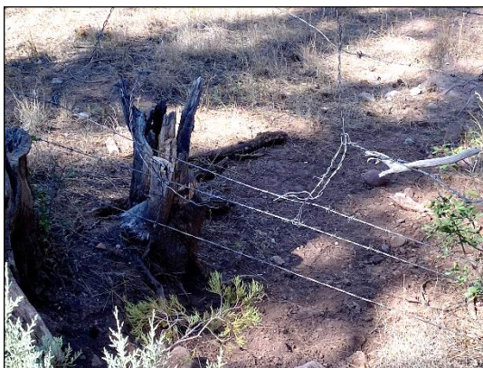
Figure 3- 91. Kohls Ranch section retrofit fence (left) where elk have created a “hole” in the strands though which they walk; note the smooth, bottom strand allowing animals to crawl under the fence (left), also prevalent on the Little Green Valley Section fence (right).
