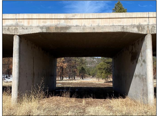
Figure 3- 99. SR 64 Cataract Canyon bridge located at MP 187.3 (left) and an individual barrel (right) suitable for accommodating elk and mule deer passage with wildlife fencing.
