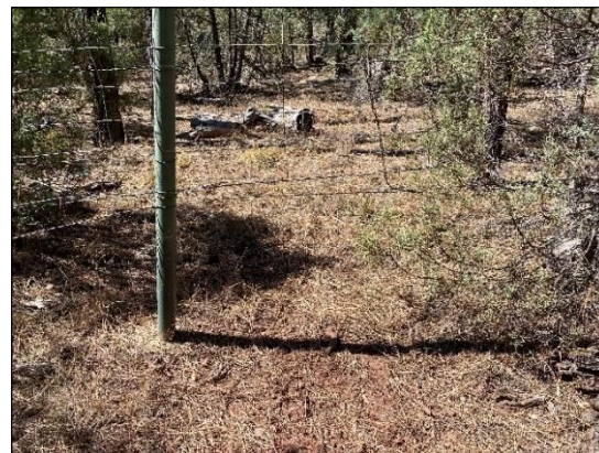
Figure 3- 91. Kohls Ranch section retrofit fence (left) where elk have created a “hole” in the strands though which they walk; note the smooth, bottom strand allowing animals to crawl under the fence (left), also prevalent on the Little Green Valley Section fence (right).
